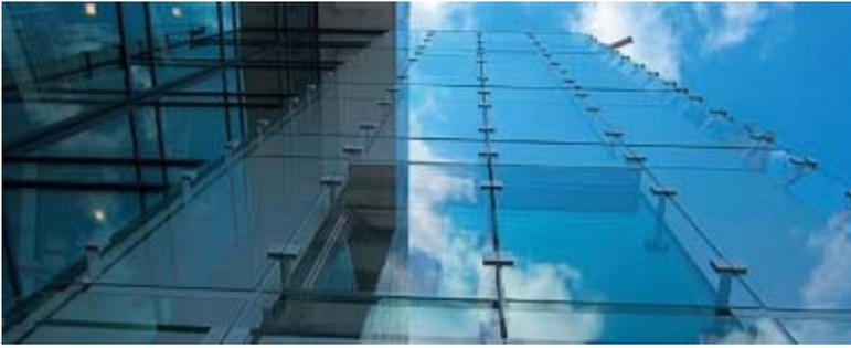
*The 12 floor, 189,700 sqft building exploits the highly transparent characteristics of SentryGlas® to compliment the low-iron glass used in the weather shield on all aspects of the building.*
