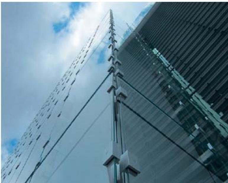
*Unlike typical structural wall systems, the edges are totally exposed, so the architects and installers had to be confident*
